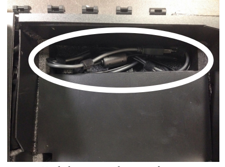
Cables under printer
